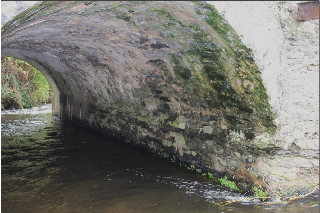
Plate 9: Detail of pier between southern two arches from east opening. Note extension of archway to west by approximately 50% in cast concrete.
