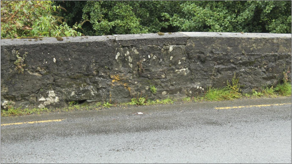
Plate 3: Road-side detail of original, eastern parapet masonry to crown of bridge. Note drainage hole from bridge deck to left of centre of photograph and original vertical coping stones beneath, or replaced by cast-concrete capping.
