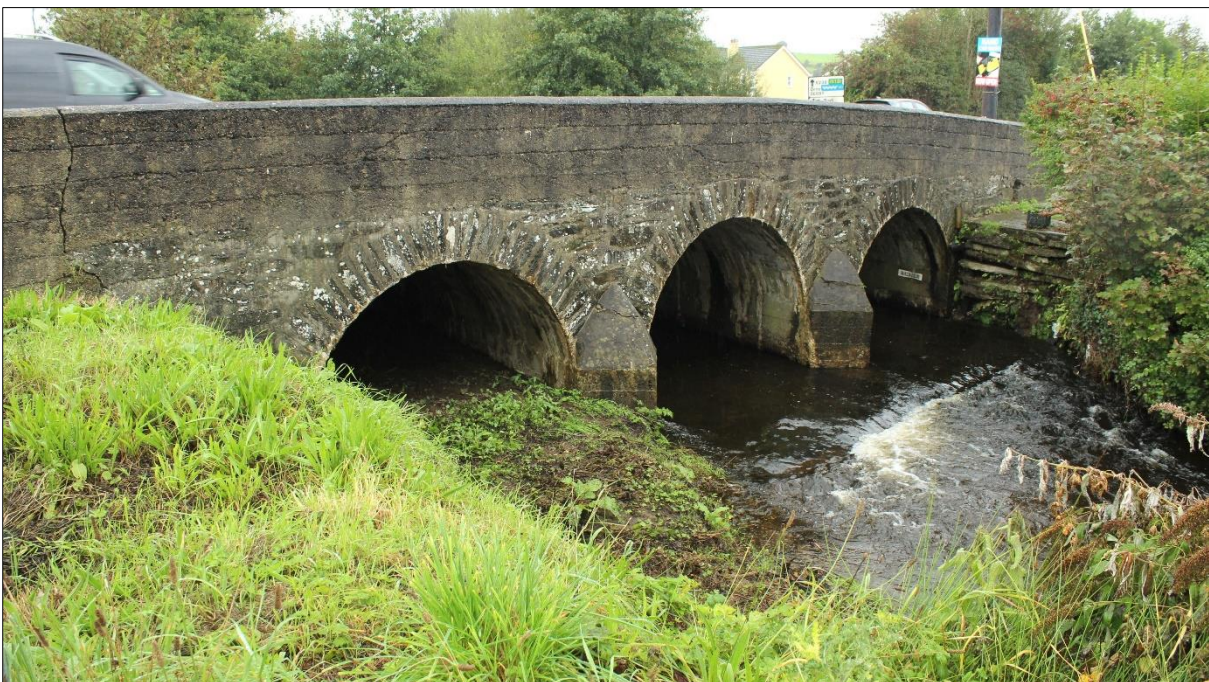
Plate 4: West elevation from north with stone arch and spandrel masonry over mid twentieth-century cast-concrete arch extensions. Parapet, cutwaters and paved river bed are also all of cast-concrete.
