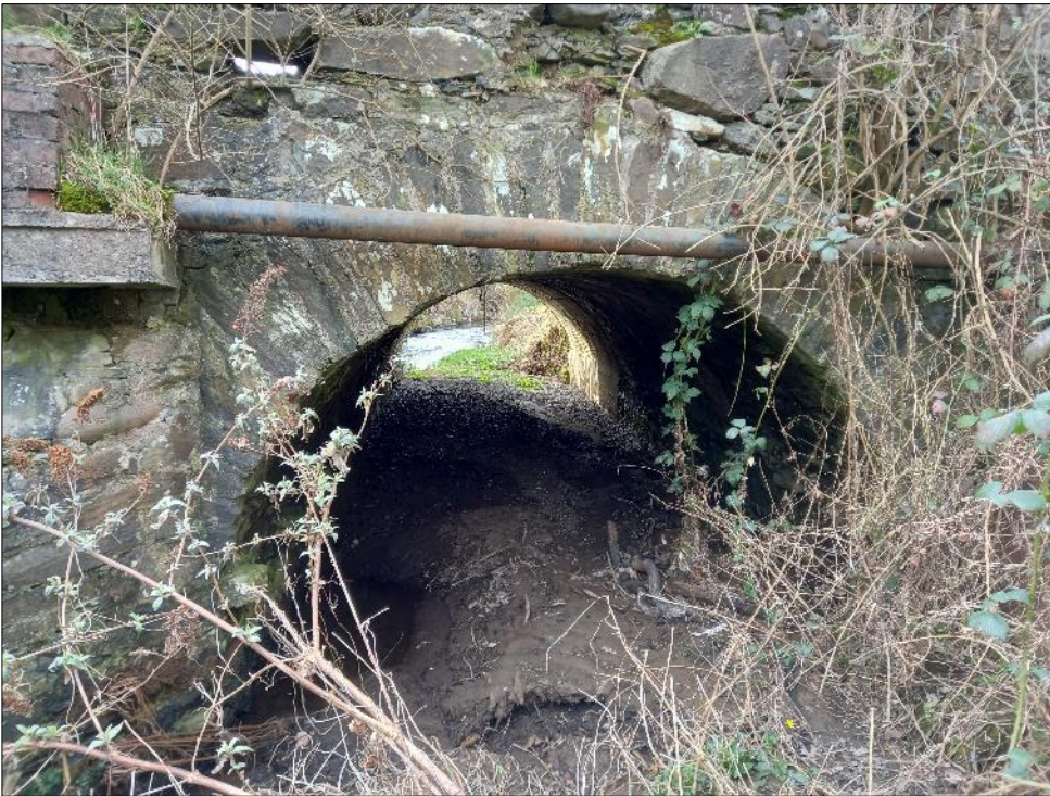
Plate 15.12: View towards west of northern silted bridge arch on eastern bridge elevation
