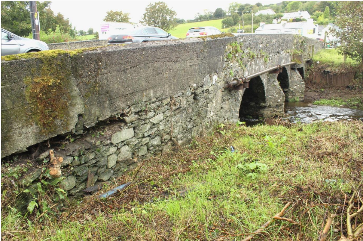
Plate 6: East elevation from south bank with cast-concrete extension to parapet masonry added when road approaches to bridge were raised during mid twentieth-century.
