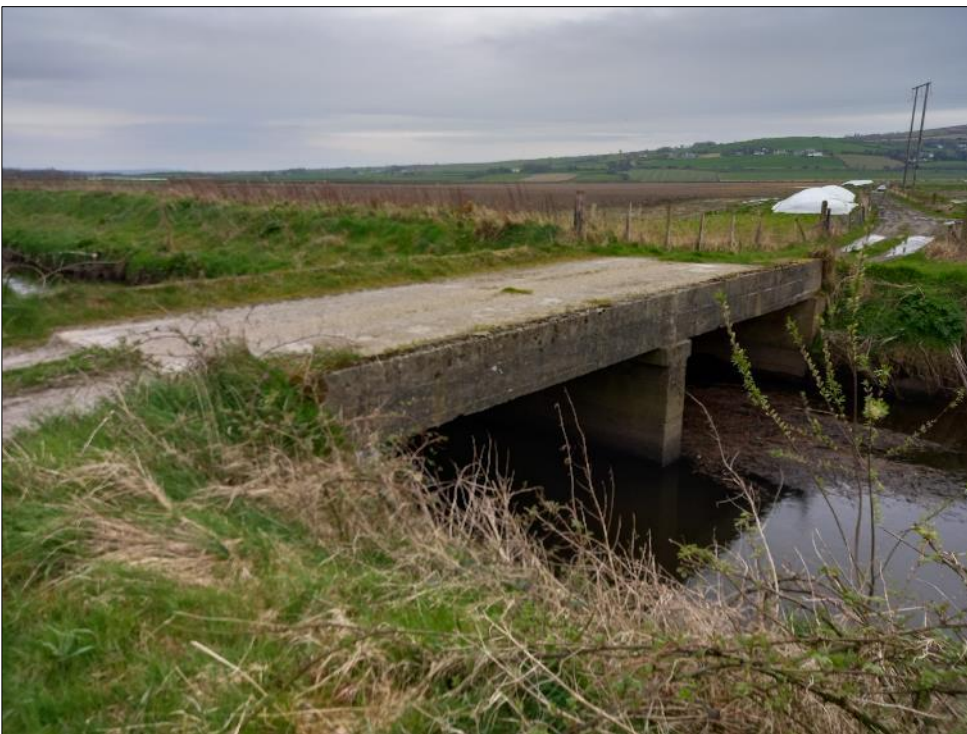
Plate 15.28: View towards southwest of concrete vehicular bridge crossing the Skeoge River
