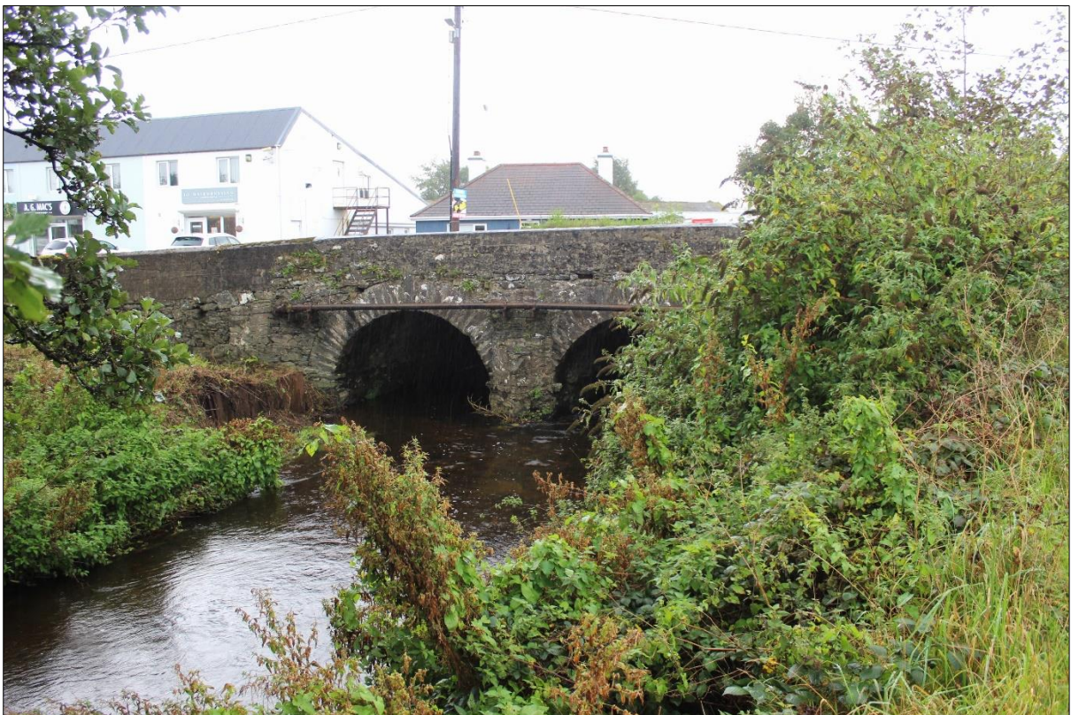
Plate 10: Original east elevation from north bank
