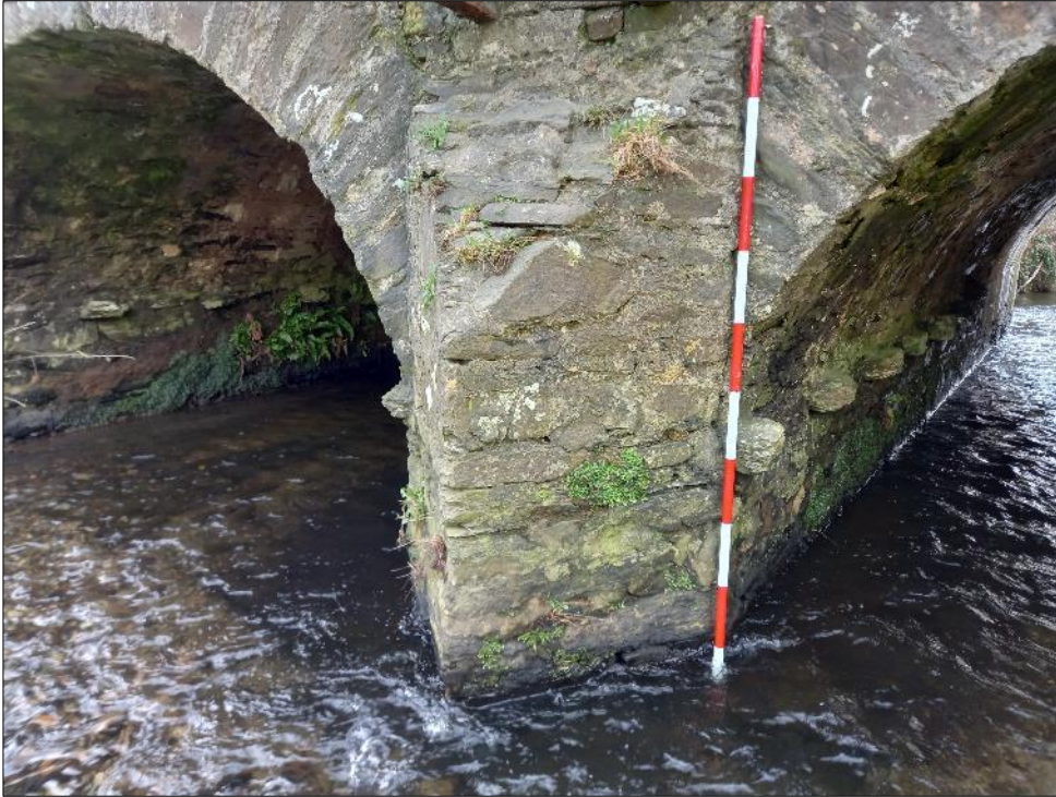
Plate 15.13: View of eastern bridge elevation and stone rubble-built cutwaters and voussoirs
