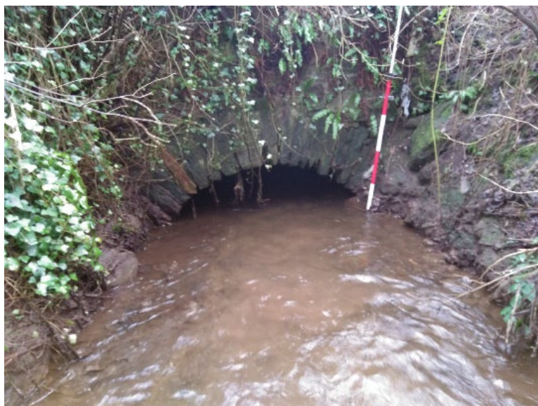
Figure 3.25: Inlet of N15 culvert upstream of CPI Centre
