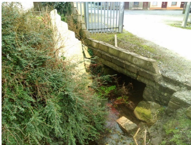
Figure 3.23: McGlynns culvert inlet
