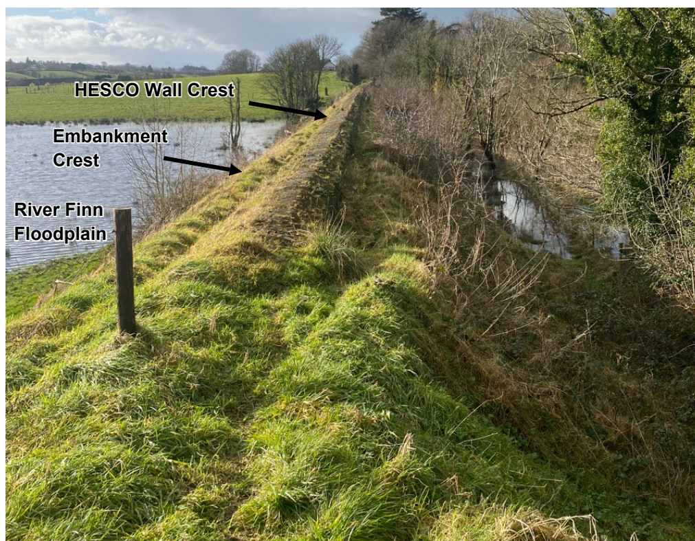
Figure 3.14: CPI Flood Defence Embankment with HESCO flood wall system lining the crest.
