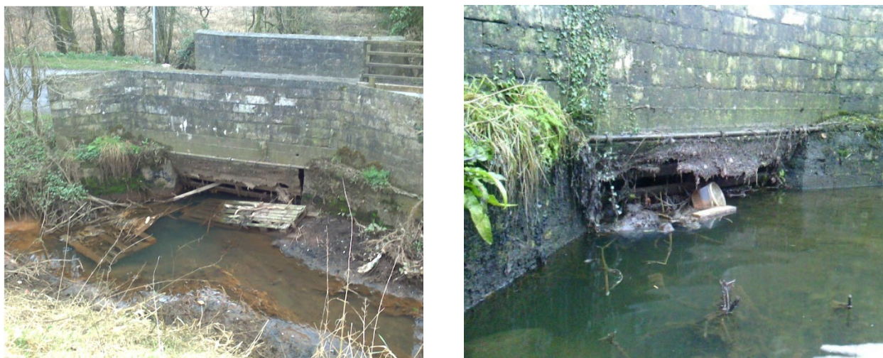
Figure 3.28: Wooden screen at downstream extent of Hollow Road Bridge
