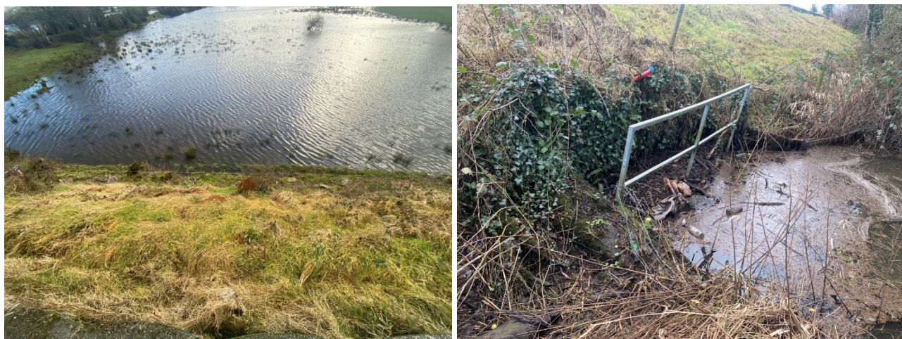
Figure 2.5: Flooding downstream (left) and upstream (right) of CPI embankment February 2021
