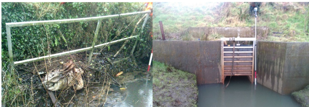
Figure 3.29: (L) CPI Embankment culvert inlet with debris screen (submerged at time of survey). (R) Sluice gate non-return and valve at downstream extent of culvert
