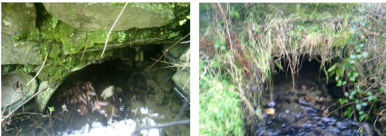
Figure 3.31: (L) South Finn double-barrelled culvert inlet. (R) Culvert outlet.
