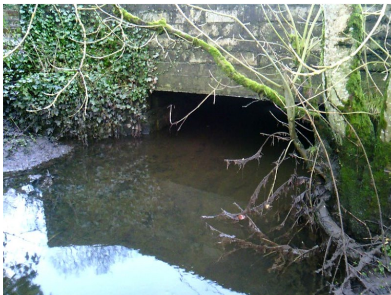
Figure 3.27: Hollow Road Bridge opening (downstream)
