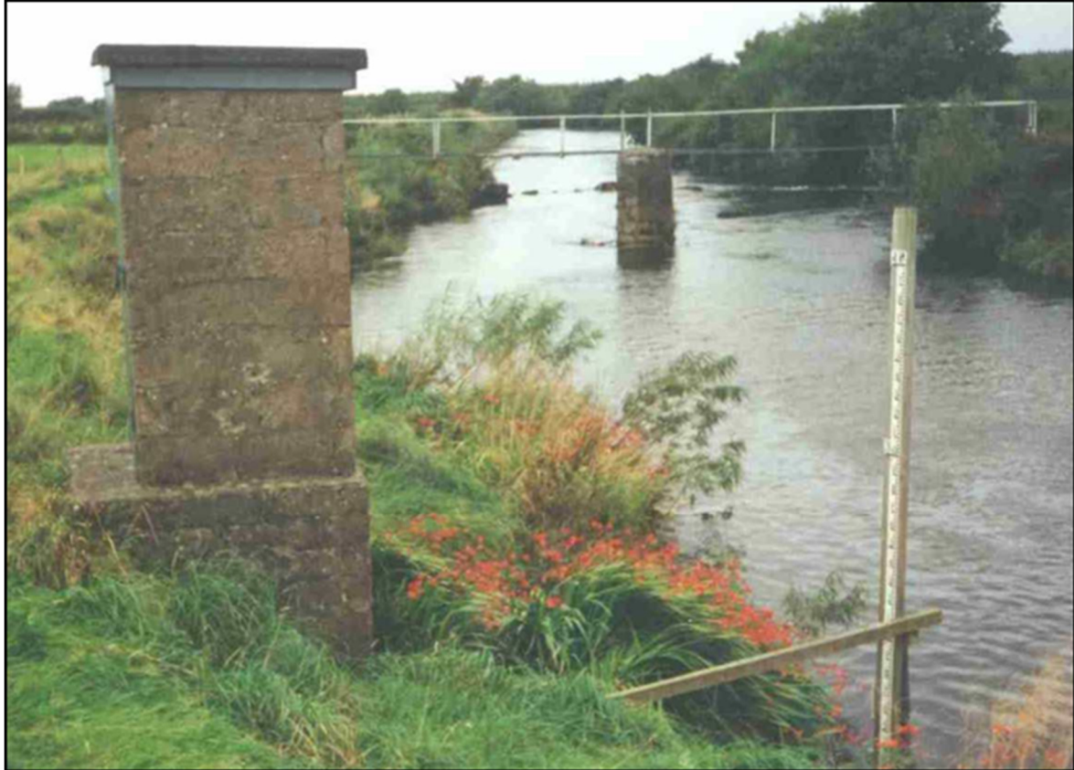
Figure 2.3 Looking downstream from Clonconwall Ford gauging station, with rudimentary footbridge and stepping-stones
