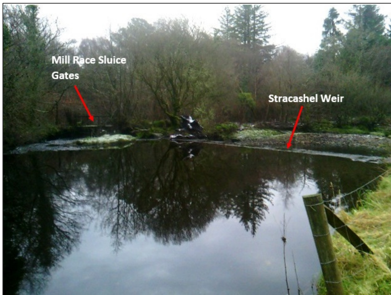
Figure 2.13 Location of the mill race sluice gates in relation to Stracashel River weir
