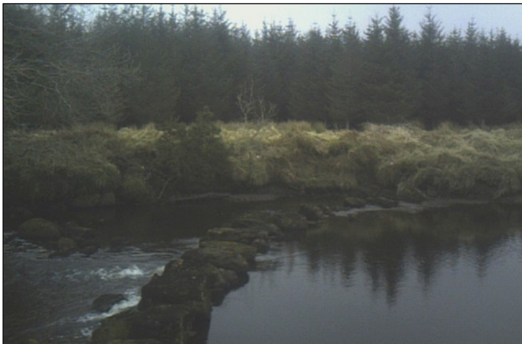
Figure 2.4 De facto weir created by stepping-stones, downstream of Clonconwall Ford gauging station
